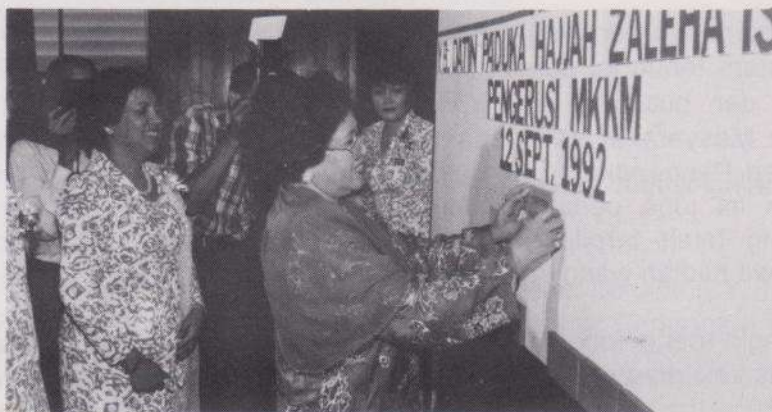
The 1st brick and the brick fund is officially launched
