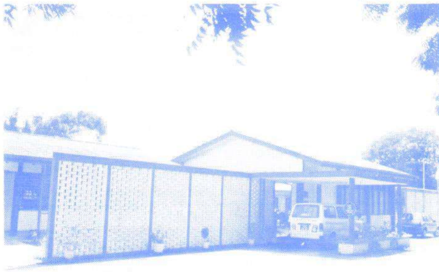
Phase I Building – Our Own Centre.
